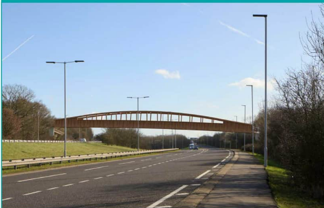
Figure 4-53: Proposed view of new bridge over the A127 to the west of J29
